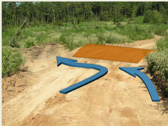
Properly constructed waterbar and outlet for dispersing water.
